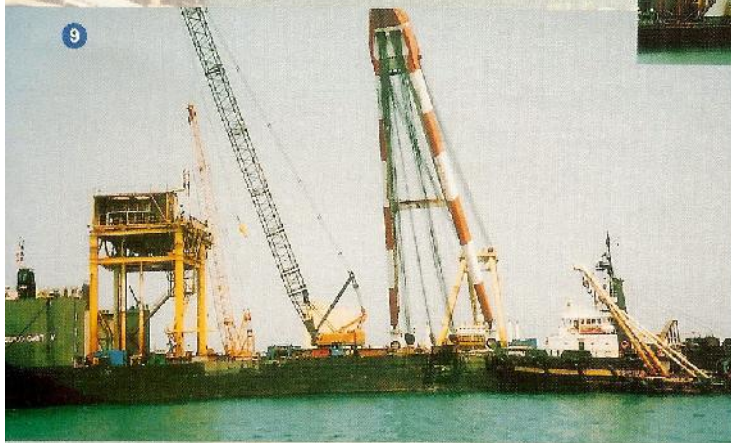
⑥ 鑽油平台拆除施工實況。 Demolishing operation of oil drilling platform.
